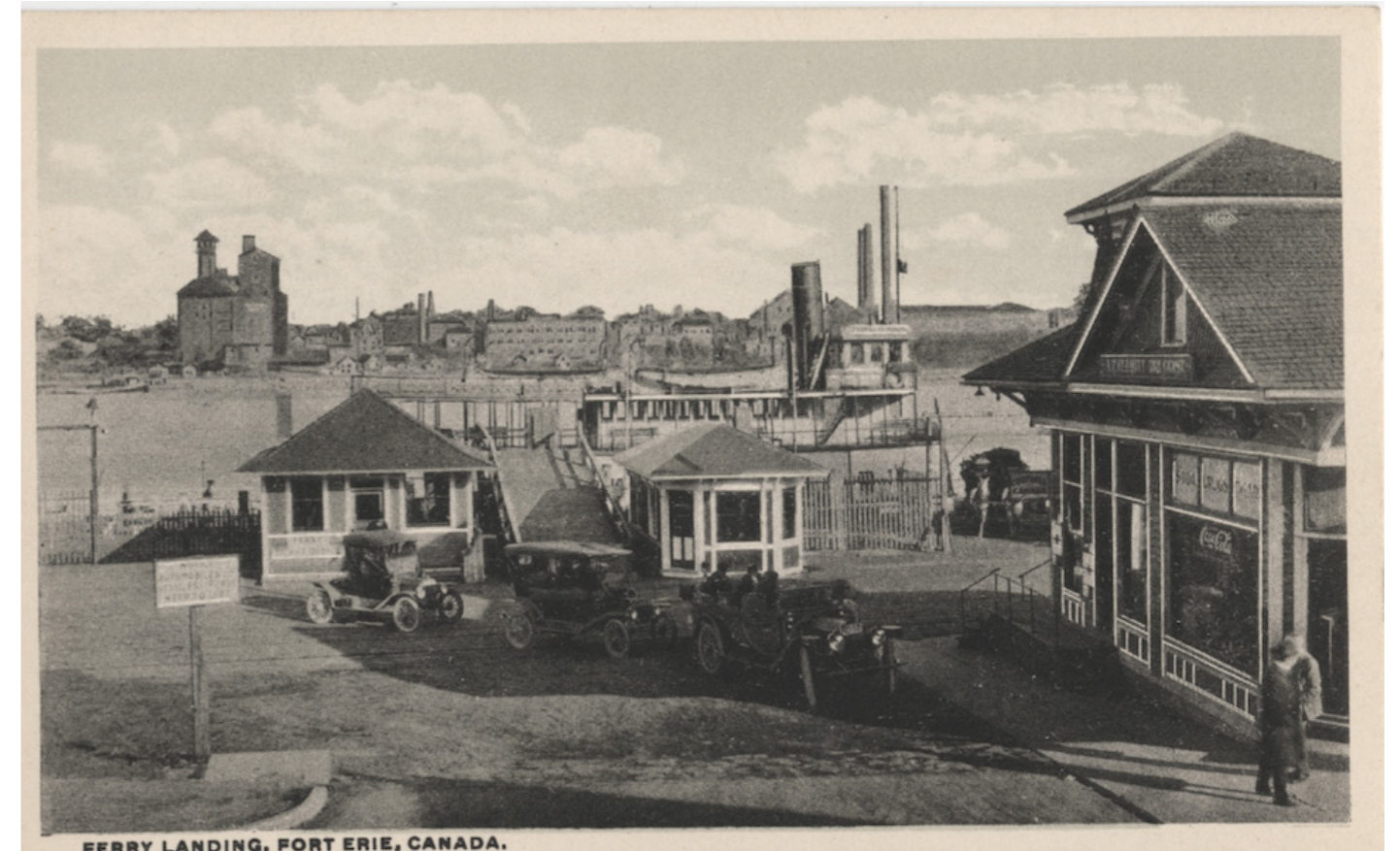
ABOVE: Ferry Landing, Fort Erie Canada around 1920
